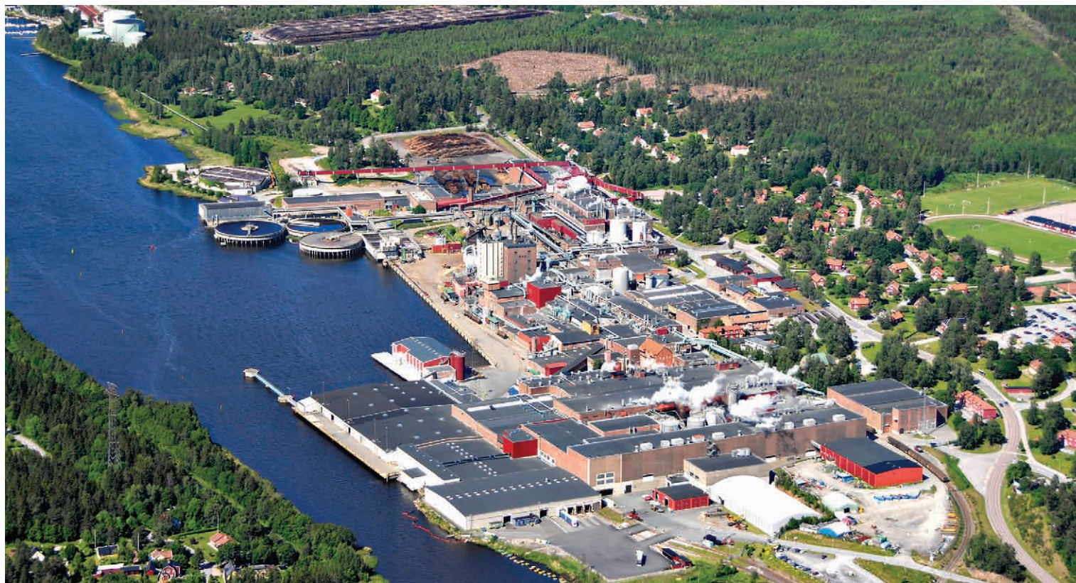
Hallsta 1. Hallsta paper mill produces 550 000 tonnes of lightweight uncoated magazine papers and book papers on two paper machines
