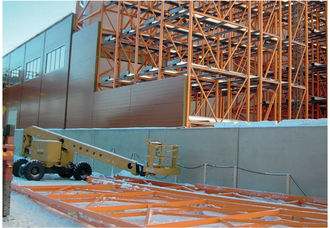
Figure 2 To save with building costs, the wall and roof elements can be attached and supported directly by the rack structure
